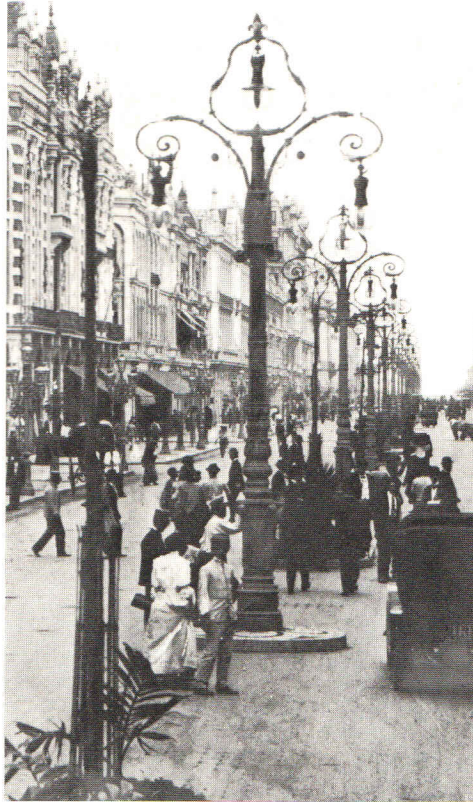
British contractors installed street lights like London's in Rio de Janeiro.
