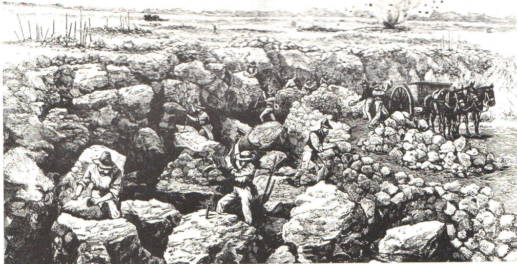
Miners blast the layers of nitrate lying three feet below the surface of the Tarapacá plateau.
